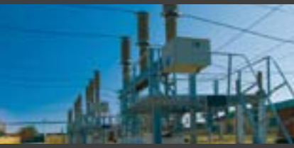
On Grid Solar Field
